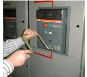
Complete closed door breaker operation
